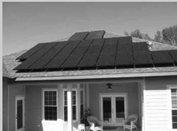
Zero energy 2250 sq. ft. home (note the solar panels on the roof) built in Gainesville, Florida by Tommy Williams in conjunction with the Florida Solar Energy Institute (FSEC); for more information, see reference #4.
